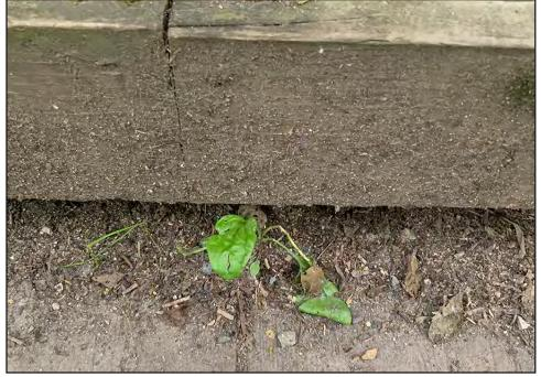
This little "weed" indicates that Bridge Four could use a good cleanup. This bridge and Bridge Five have flat decks and thus do not flush themselves clean when it rains – unlike the other bridges which are arched. This results in a buildup of soil and vegetative matter in which seeds can take root. Perhaps this could lead to decay of the bridge deck as well.
